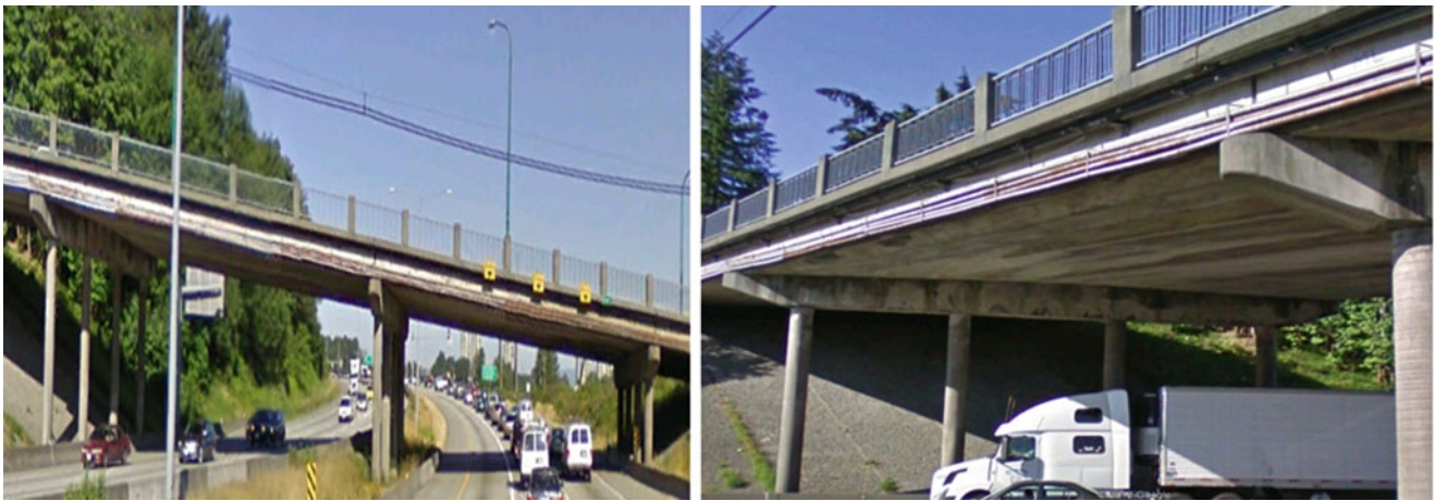
Fig. 15.5 Douglas road underpass (Douglas Rd)
