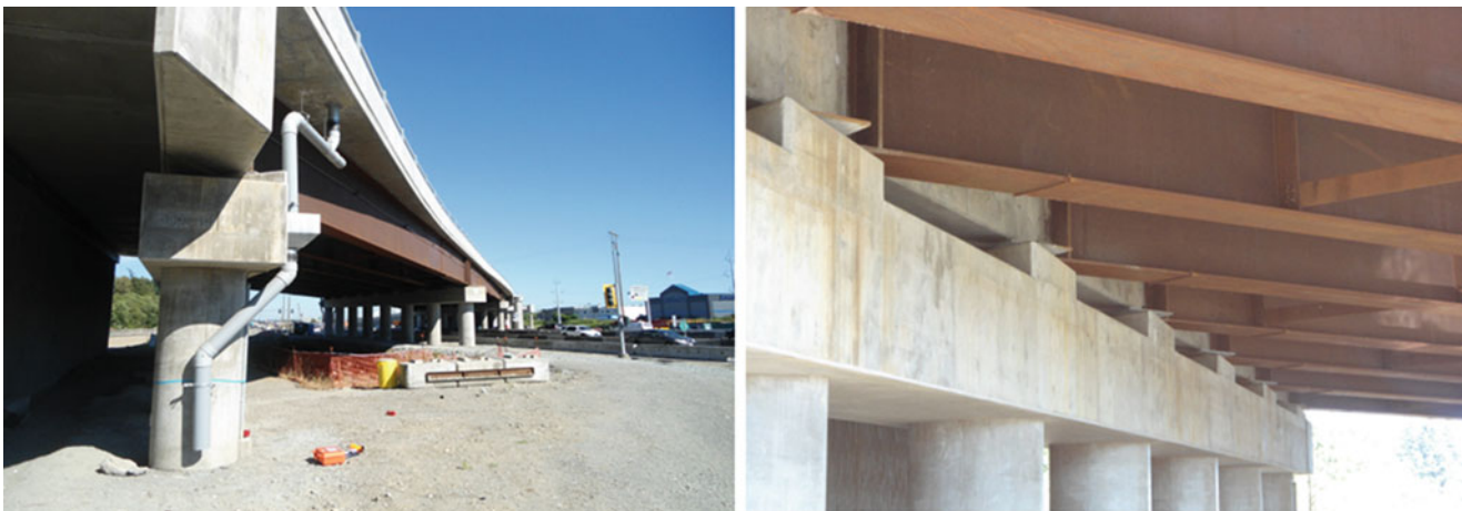
Fig. 15.4 Highway 1 and Lougheed highway underpass (LHH-EB underpass)
