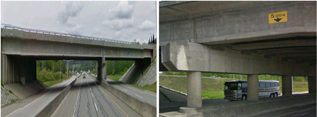
Fig. 15.3 Annacis highway and Highway 10 underpass (HWY 10th)
