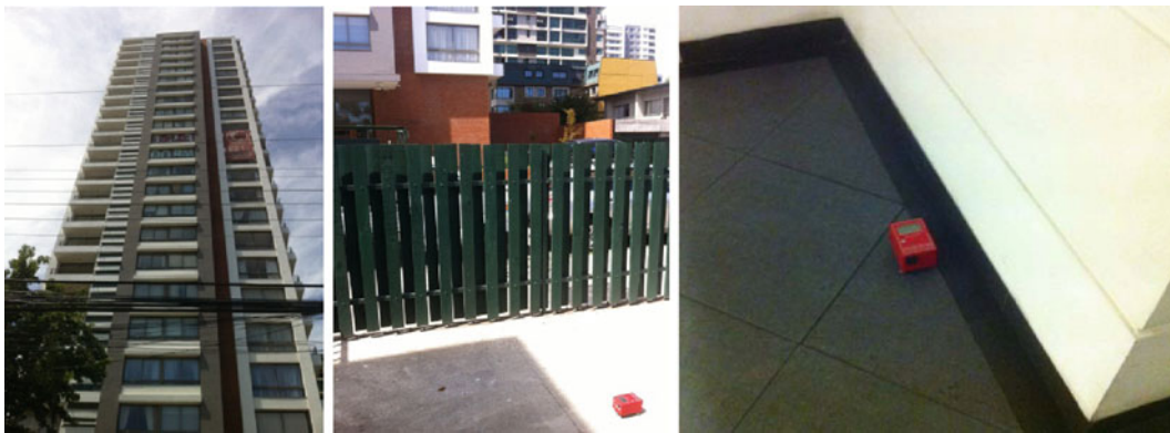
Fig. 14.5 Elevation of 24 Storey Building and ambient vibration measurements
