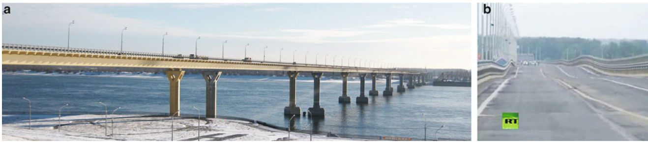
Fig. 10.1 Volgograd Bridge (photo: J. Distl) (a) and its vibrations in May, 2010 (source: RT news channel at youtube.com) (b)
